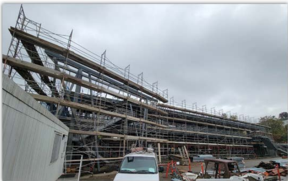
BUILDING H SOUTH FAÇADE PROGRESS
